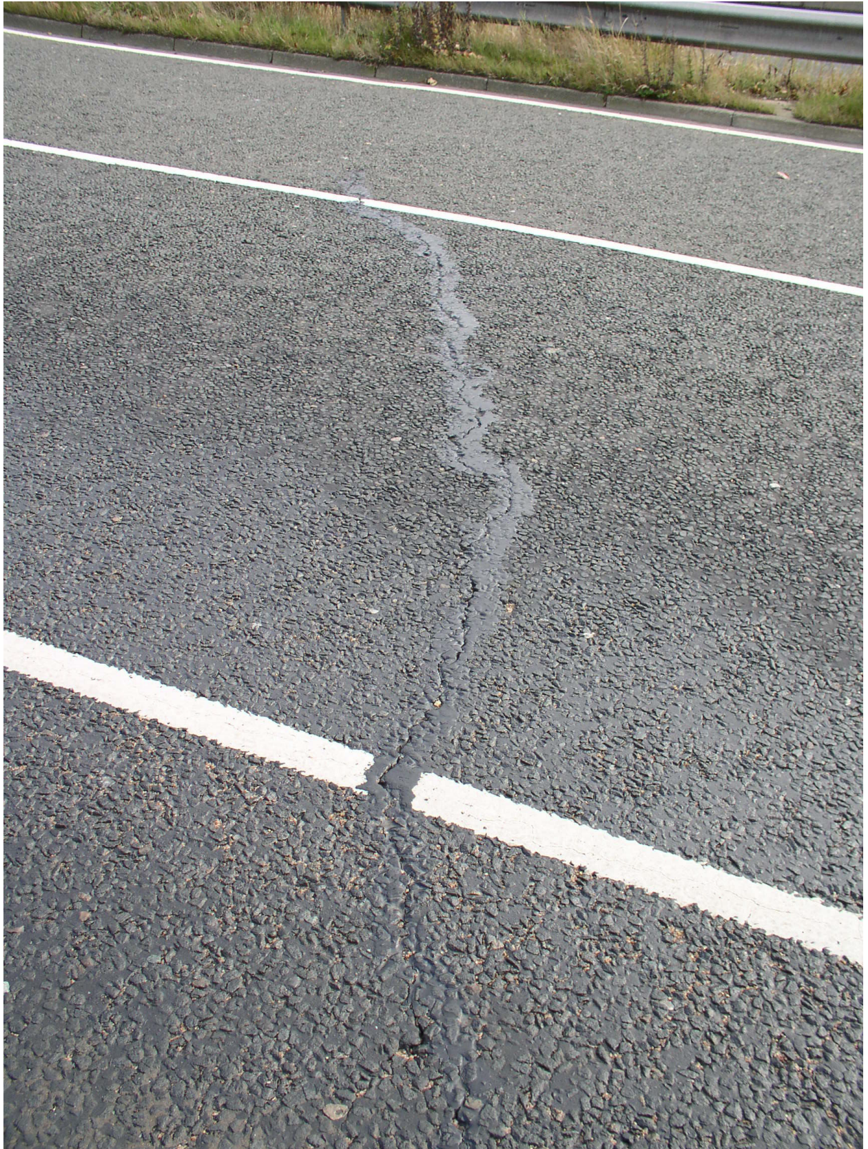
Figure 4 Fissure seen in the surface of the northbound carriageway of the A690, note that the fissure is not a perfectly linear feature. This is feature H shown in Figure 9.
